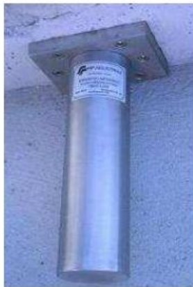
Seismic retrofit of the Basilica of San Francesco in Assisi: particular of the SMA devices.
