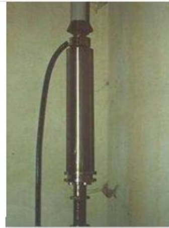
Seismic retrofit of the bell tower of the church of San Giorgio in Trignano: (left) elevation of the structure and (right) particular of the SMA rod used.
