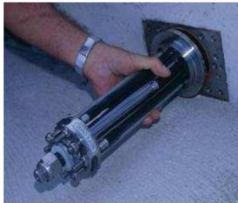
Seismic retrofit of the Basilica of San Francesco in Assisi: particular of the SMA devices.
